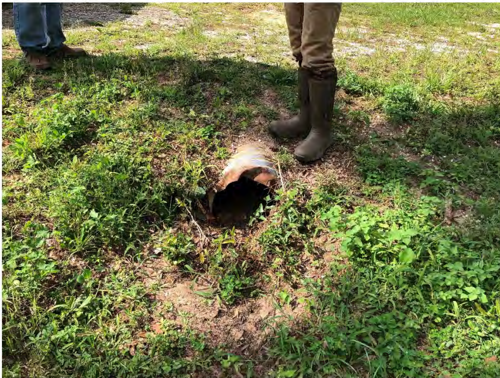
Figure 9252: Photo taken facing North toward P-CO-15 along Pecan Grove St.
