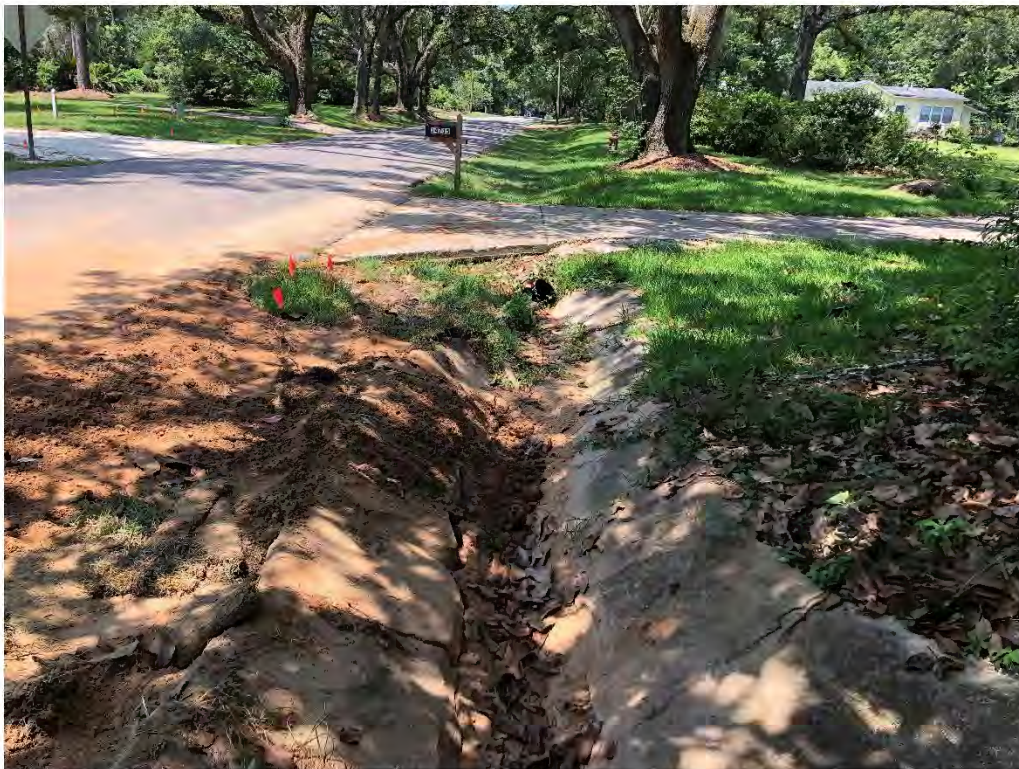
Figure 9660: Photo taken facing SW toward a concrete ditch that is full of dirt along Oak St.
