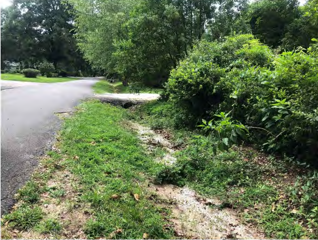
Figure 9183: Photo taken facing North toward BB-CH-8 along Bay St.
