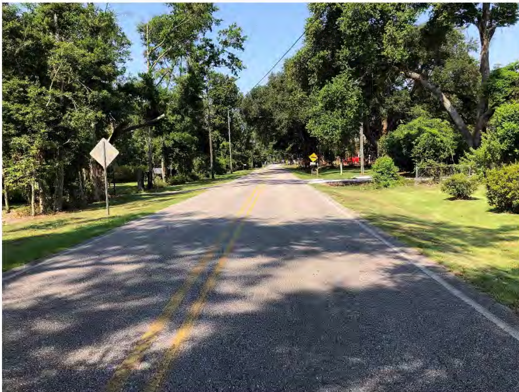
Figure 9566: Photo taken facing West of MN-CH-14 along Gates Ave.
