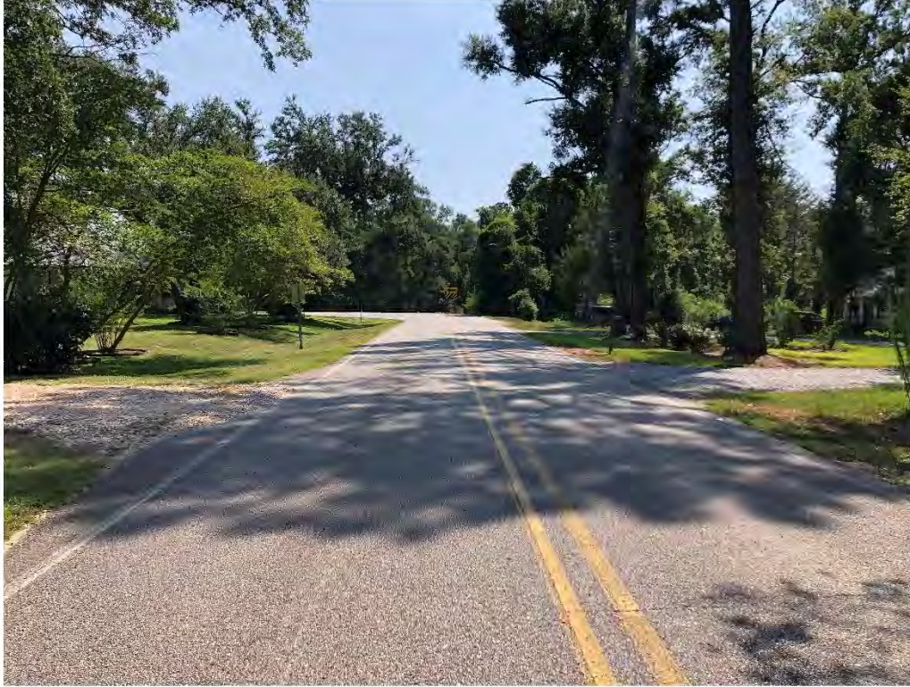
Figure 9567: Photo taken facing West of MN-CH-12 along Gates Ave.
