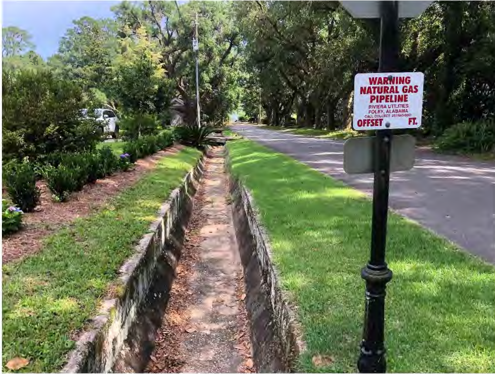
Figure 9230: Photo taken facing South toward CH-200 along Jessamine St.
