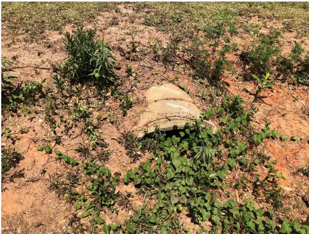
Figure 9624: Photo taken facing North toward a very silted OAK-CO-7 across Jessamine St.
