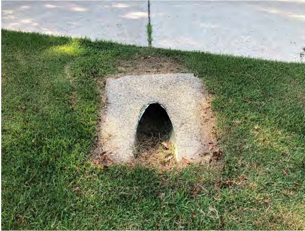
Figure 9492: Photo taken facing SE toward VG-CO-3 at the intersection of Village Green Drive and a residential driveway.
