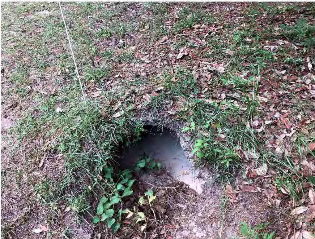
Figure 9698: Photo taken facing North toward MS-CO-2 along HWY 49.
