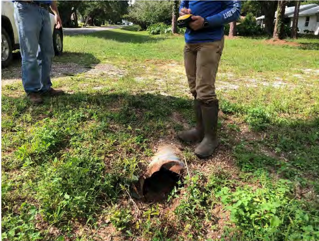
Figure 9253: Photo taken facing North toward P-CO-15 along Pecan Grove St.
