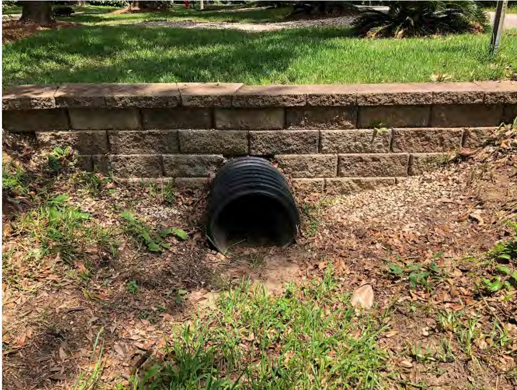
Figure 9129: Photo taken facing East toward P-CO-22 along Oak St.
