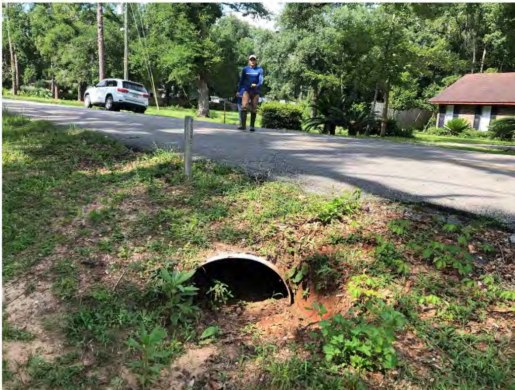
Figure 9242: Photo taken facing SW toward a silted P-CO-17 along Pecan Grove St.
