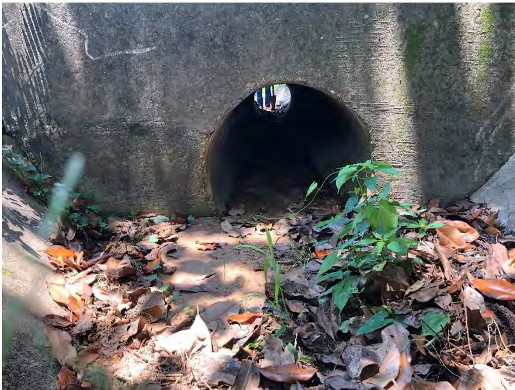
Figure 9667: Photo taken facing SW toward OAK-CO-25 at the intersection of Oak St and a residential driveway.
