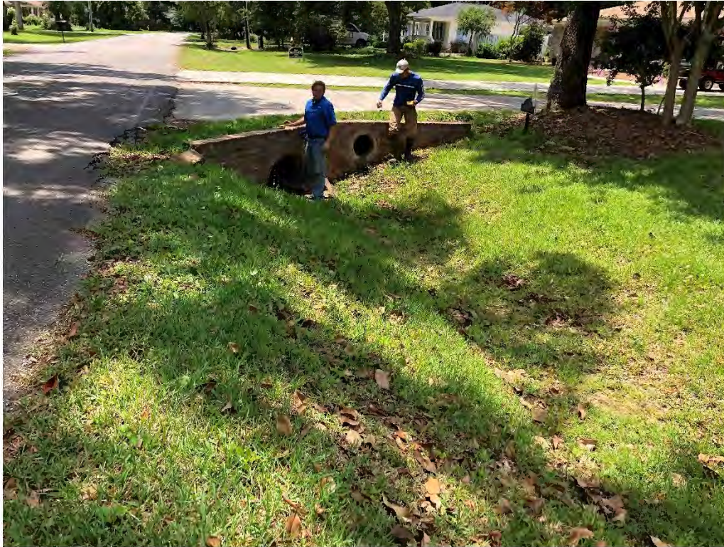
Figure 9107: Photo taken facing West toward the brick headwall with two culverts (P-CO-28 and P-CO-27) along Oak St.
