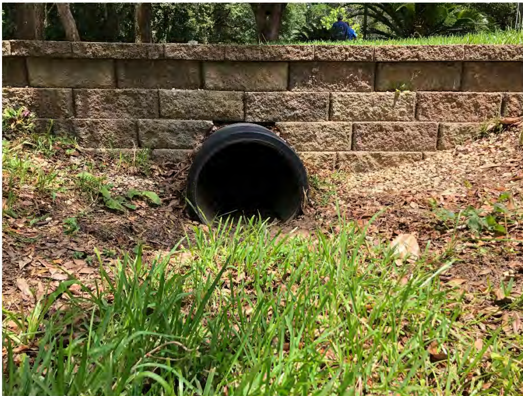
Figure 9130: Photo taken facing East toward P-CO-22 along Oak St.
