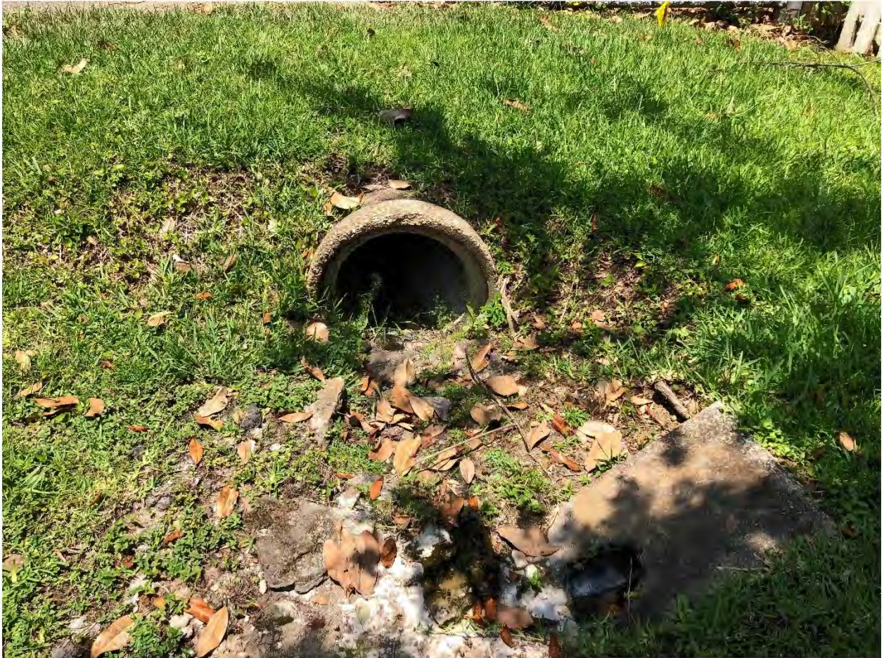
Figure 9673: Photo taken of a silted OAK-CO-26 at the intersection of Oak St and a residential driveway.
