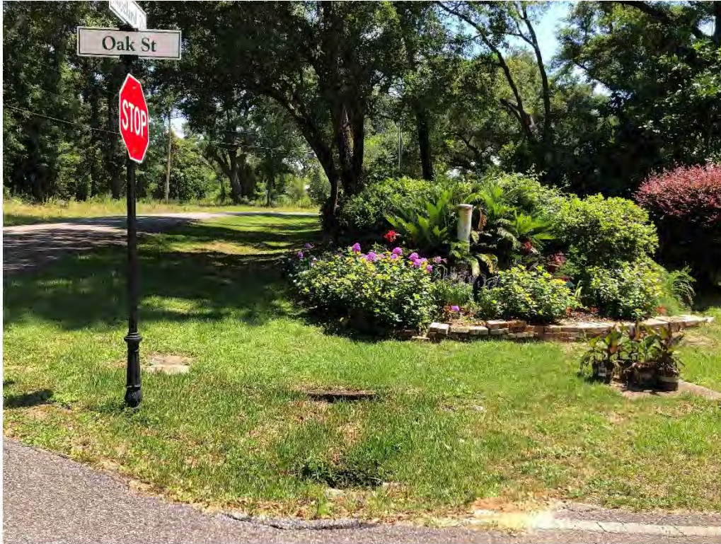
Figure 9047: Photo taken facing North toward a grassed W-CH-1 at the intersection of Woodland Ave and Oak St.
