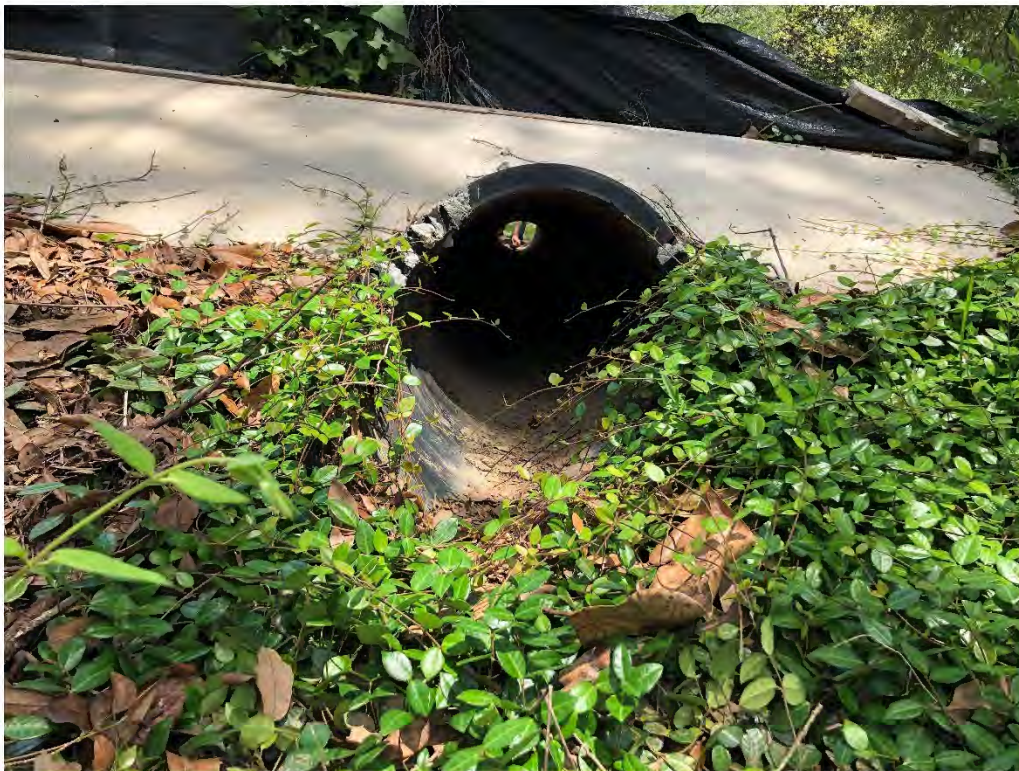
Figure 9125: Photo taken facing East toward a slightly silted P-CO-23 along Oak St.
