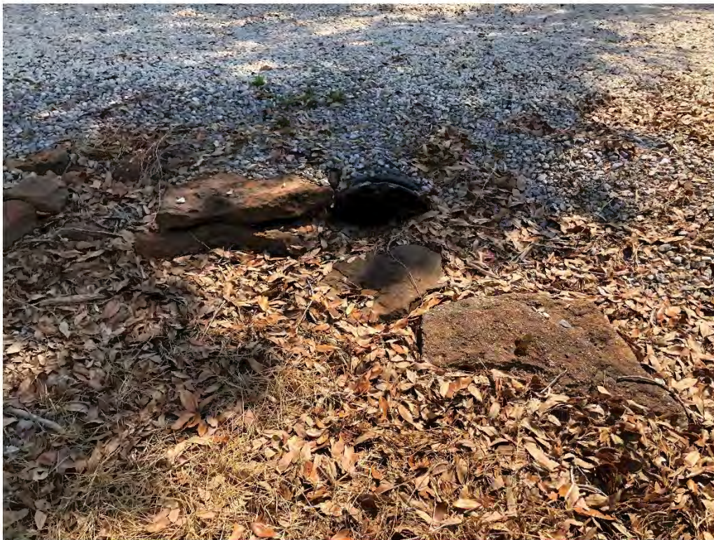
Figure 9568: Photo taken facing East of MN-CO-12 at the intersection of Gates Ave and a driveway.
