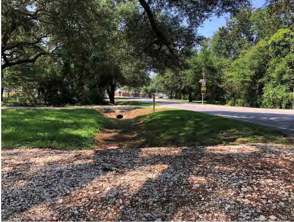
Figure 9611: Photo taken facing South toward MN-CH-7 at the intersection HWY 49 and a driveway.
