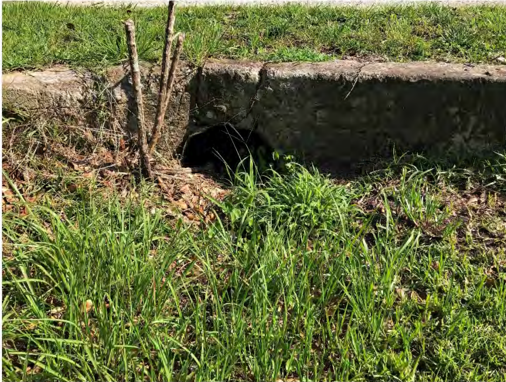
Figure 9321: Photo taken facing North toward OAK-CO-20 along Pecan Grove St.
