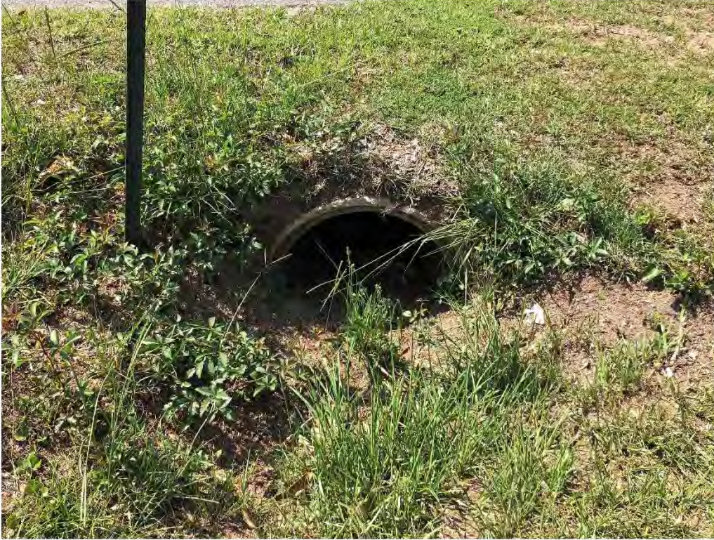
Figure 9580: Photo taken facing South of MN-CO-16 across Gates Ave.
