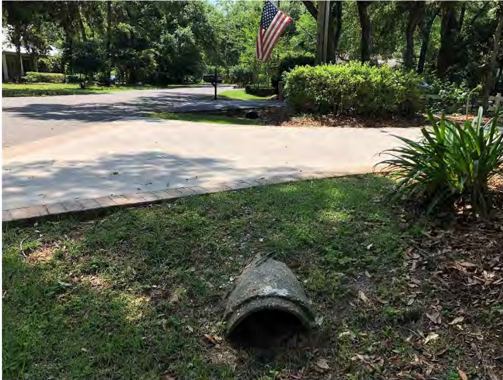
Figure 9063: Photo taken facing East toward P-CO-30 along Oak St.
