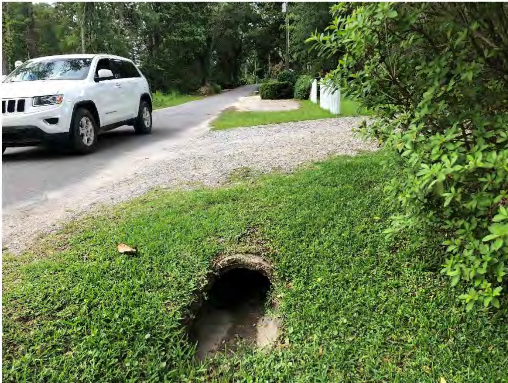
Figure 9154: Photo taken facing NE toward a silted BB-CO-14 along Island Ave.
