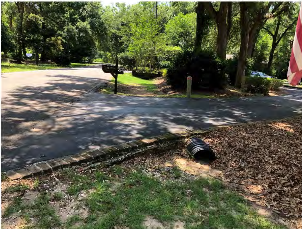
Figure 9064: Photo taken facing East toward P-CO-31 along Oak St.
