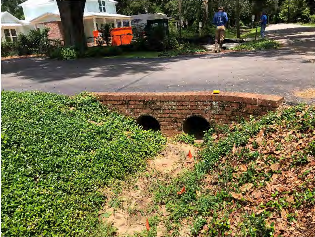
Figure 9118: Photo taken facing East toward P-CO-24 along Oak St.
