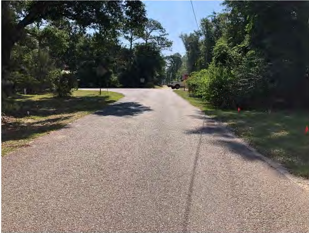
Figure 9519: Photo taken facing East toward a ditch at the intersection of HWY 49 and Cotton Stocking Lane.
