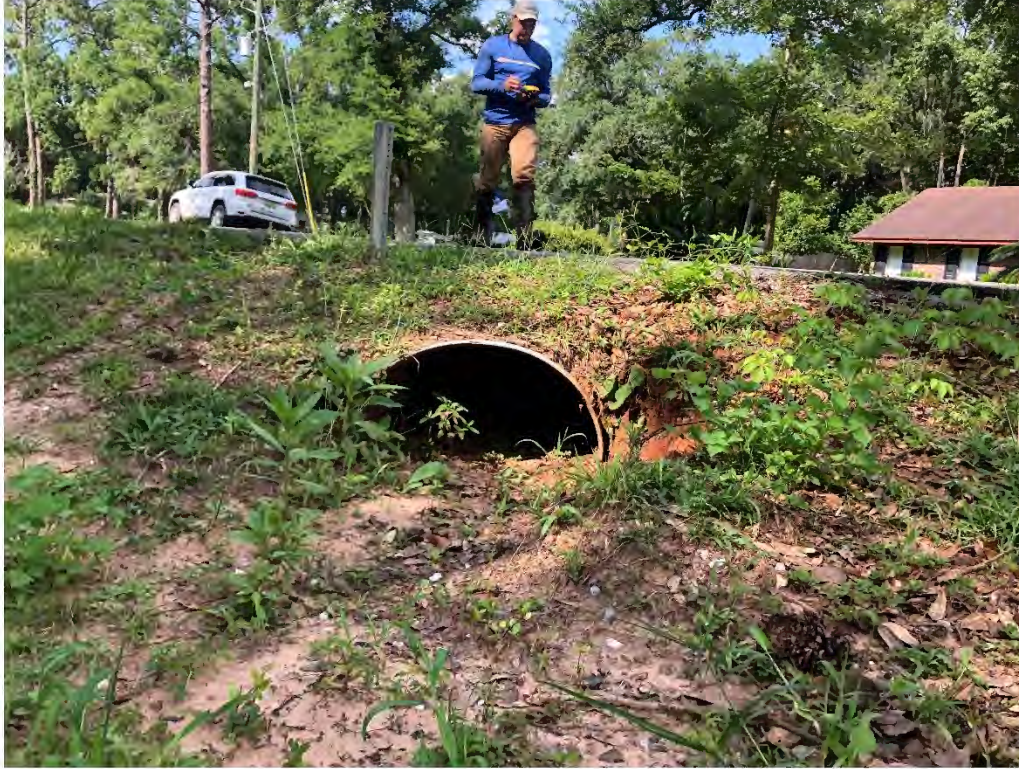
Figure 9243: Photo taken facing SW toward a silted P-CO-17 along Pecan Grove St.
