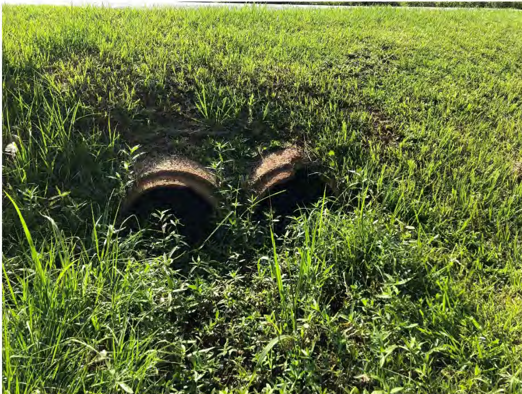
Figure 9315: Photo taken facing West toward OAK-CO-19 along Pecan Grove St.
