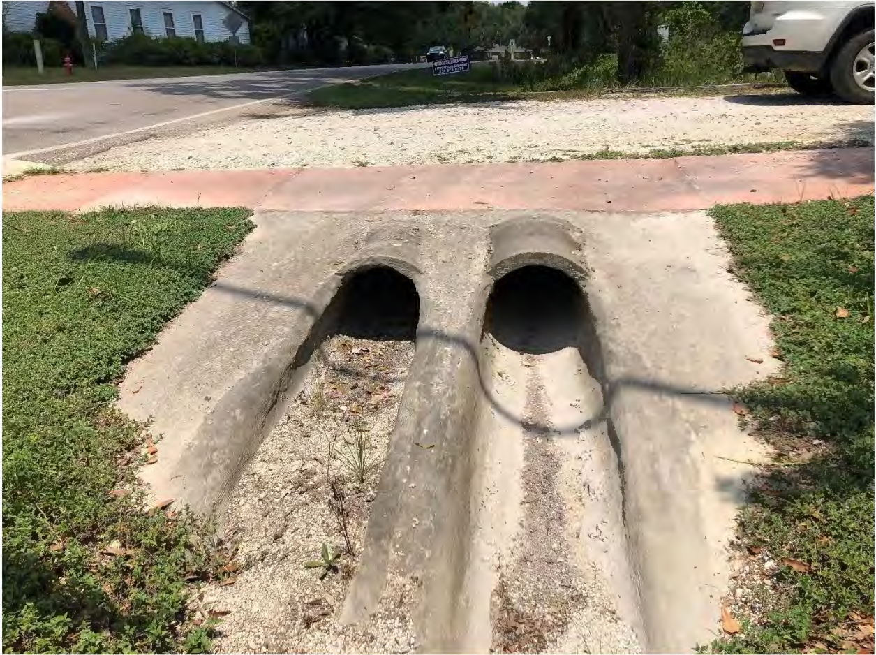
Figure 9685: Photo taken facing North toward MN-CO-17 at the intersection of HWY 49 and a driveway.
