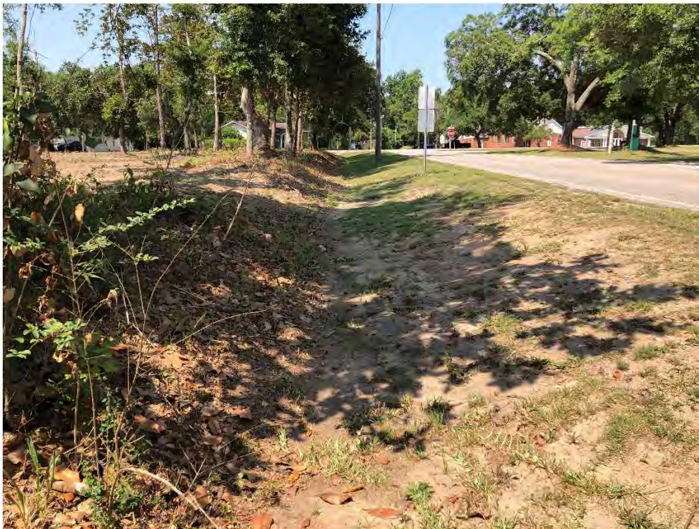
Figure 9584: Photo taken facing West of MN-CH-19 along Gates Ave.
