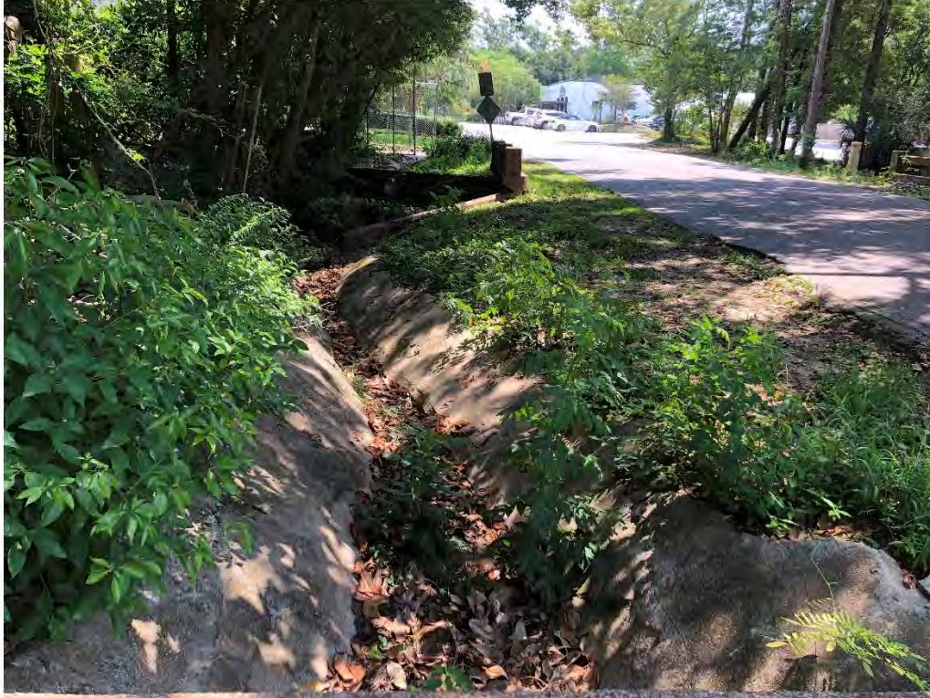
Figure 9666: Photo taken of a concrete ditch with moderate debris along Oak St.
