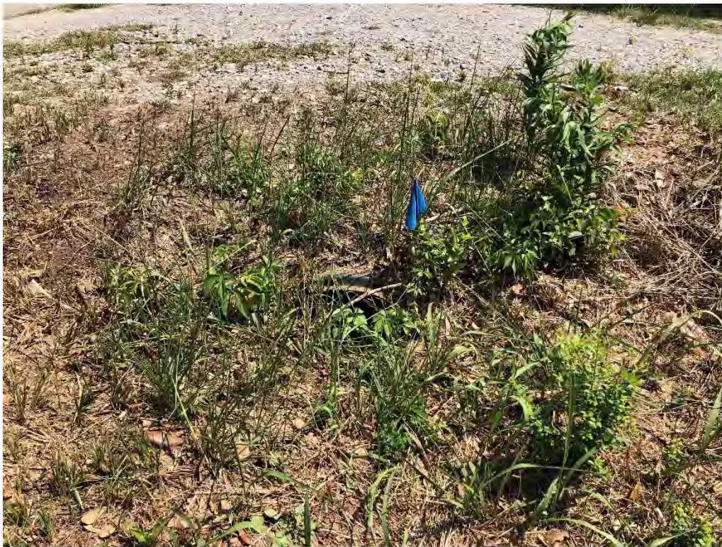
Figure 9622: Photo taken facing North toward a very silted OAK-CO-5 across Jessamine St.
