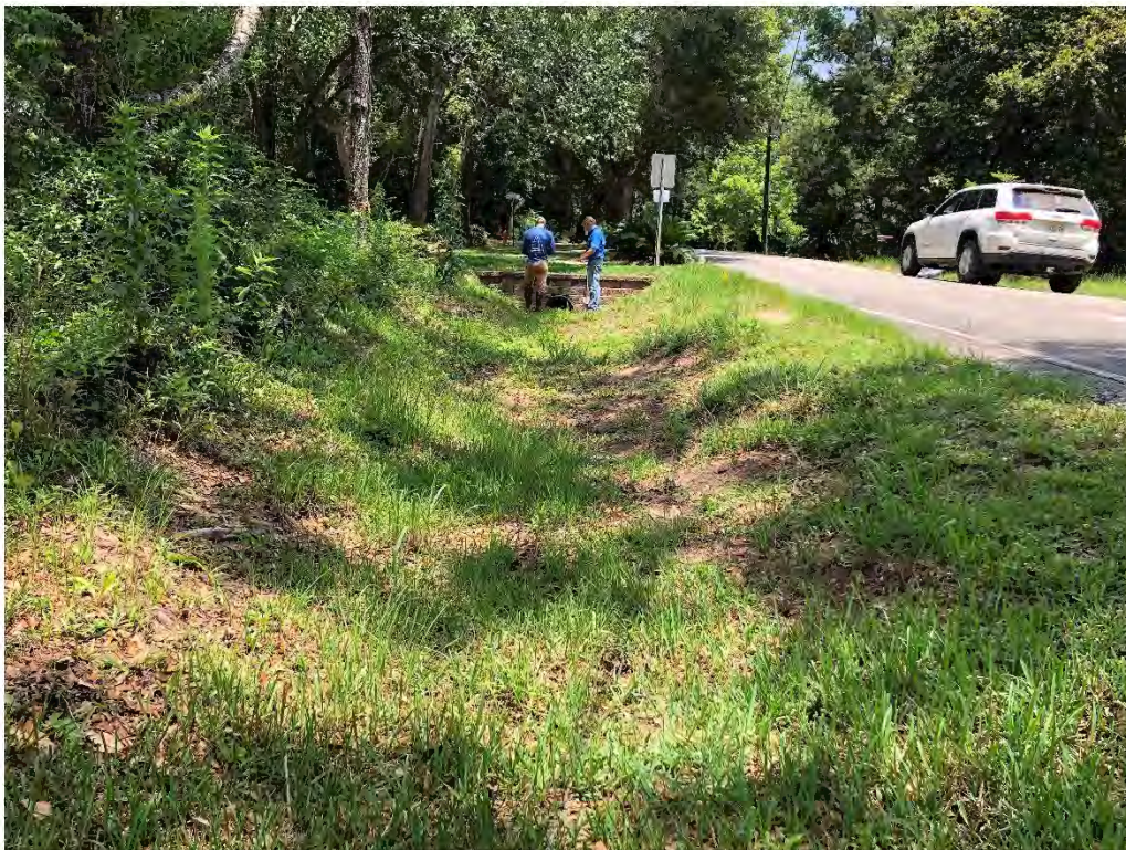
Figure 9127: Photo taken facing East toward P-CH-24 along Oak St.
