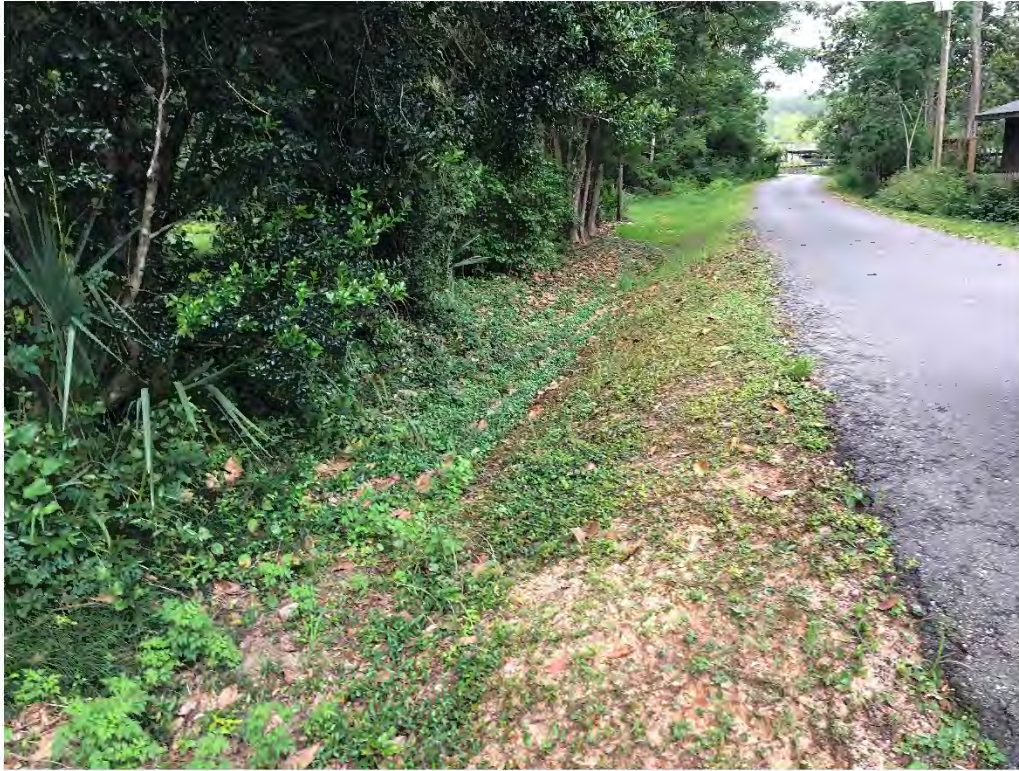
Figure 9180: Photo taken facing South toward BB-CH-12 along Bay St.
