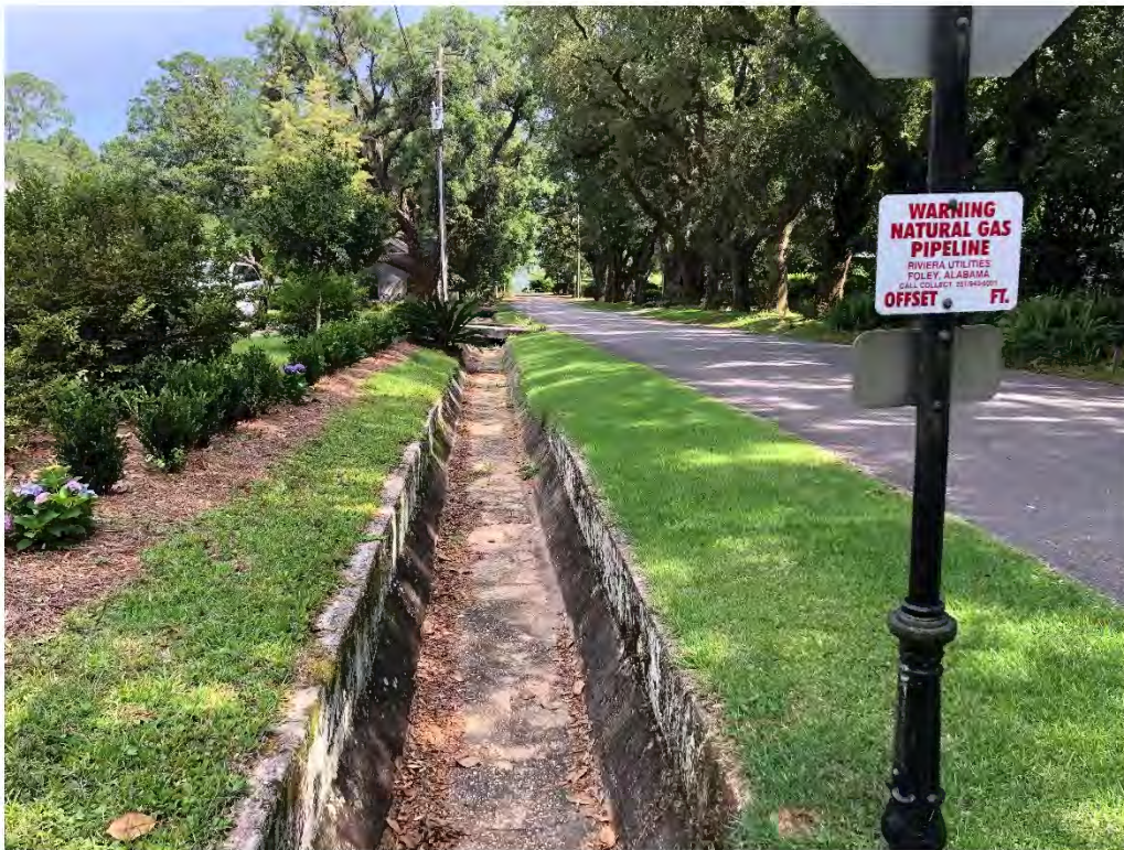
Figure 9231: Photo taken facing South toward CH-200 along Jessamine St.
