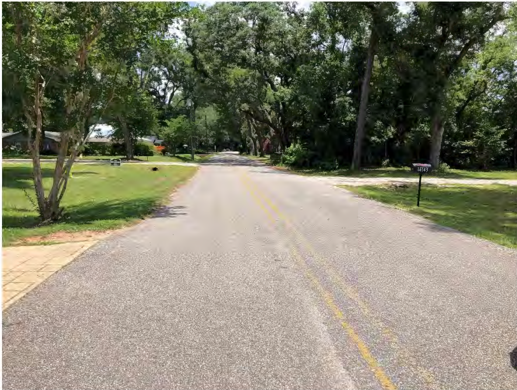
Figure 9085: Photo taken facing East toward a grassed P-CH-28 along Oak St.
