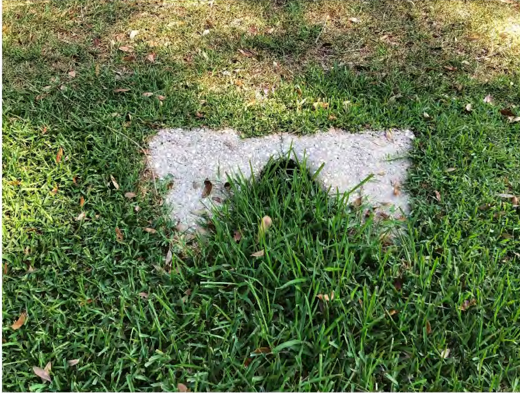
Figure 9489: Photo taken facing North toward VG-CO-2 at the intersection of Village Green Drive and a residential driveway.
