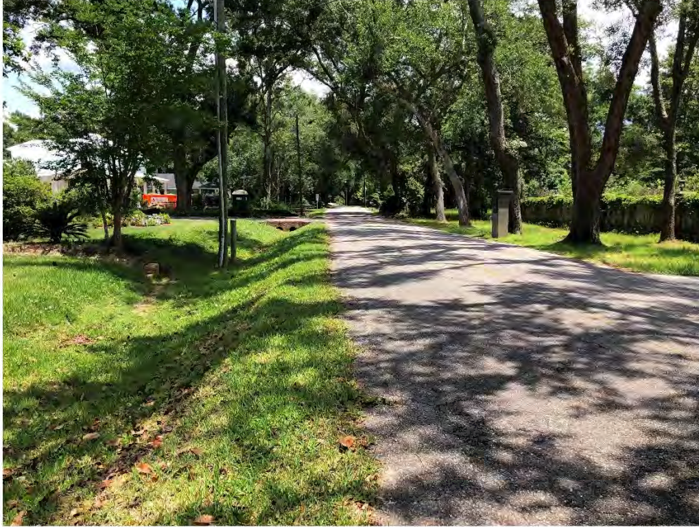
Figure 9104: Photo taken facing East toward the grassed P-CH-26 along Oak St.
