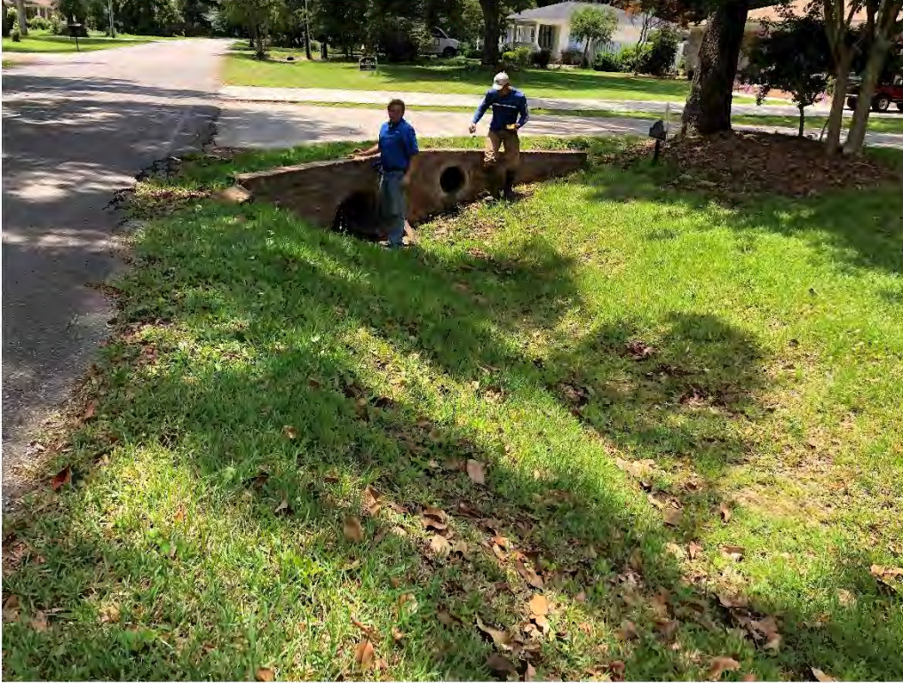
Figure 9107: Photo taken facing West toward the brick headwall with two culverts (P-CO-28 and P-CO-27) along Oak St.
