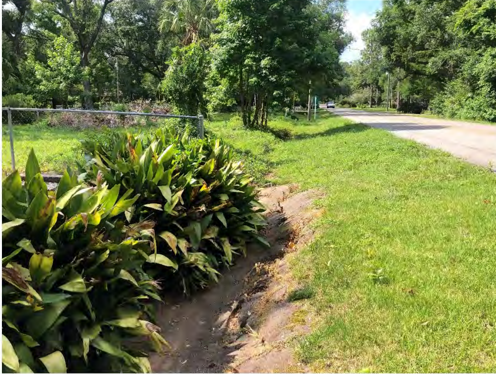
Figure 9236: Photo taken facing North toward P-CH-19 along Pecan Grove St.
