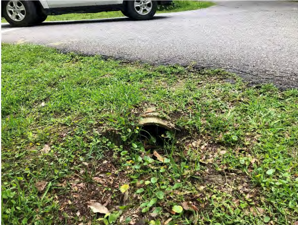
Figure 9163: Photo taken facing SW toward BB-CO-17 along Island Ave.
