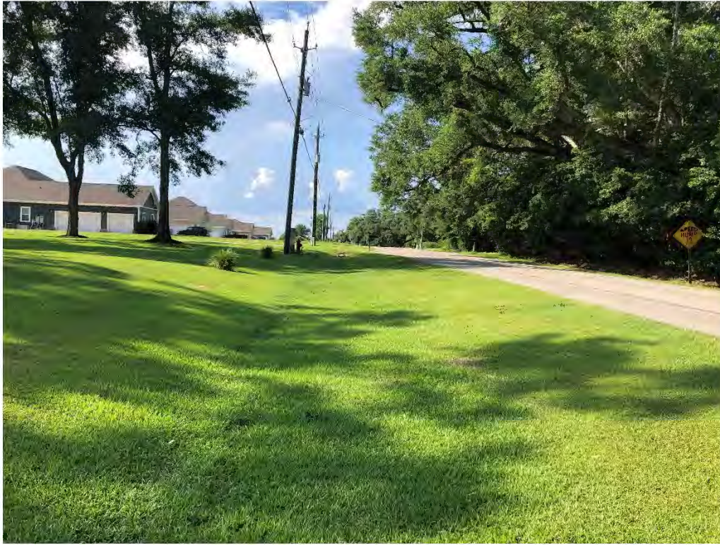
Figure 9293: Photo taken facing North toward P-CH-3 along Pecan Grove St.
