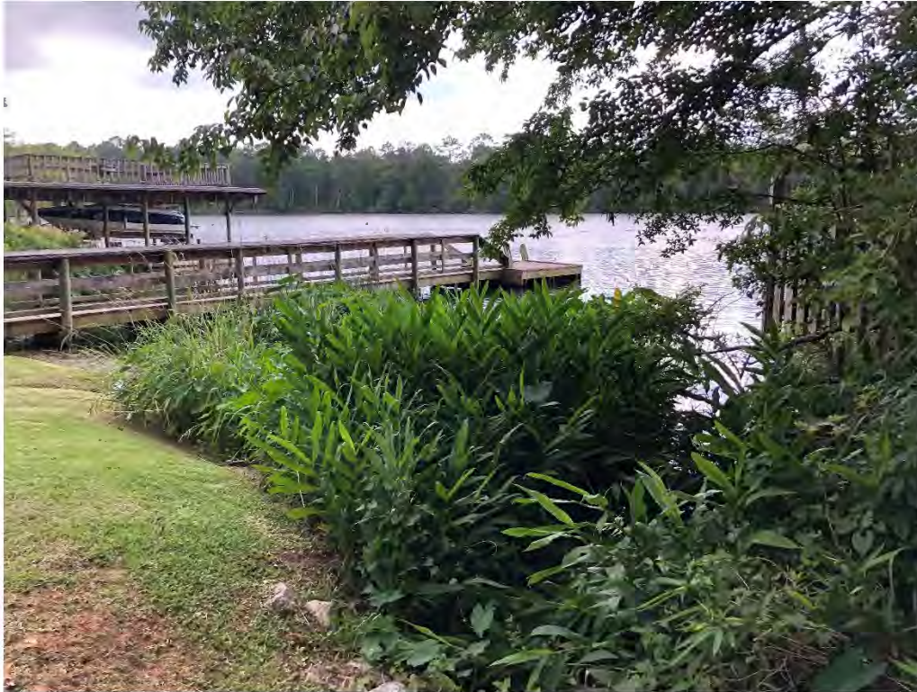
Figure 9175: Photo taken facing South toward BB-CH-13 along Bay St.
