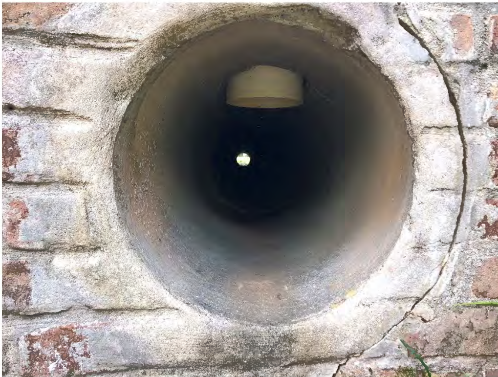
Figure 9113: Photo taken facing West toward a concrete P-CH-27 along Oak St.
