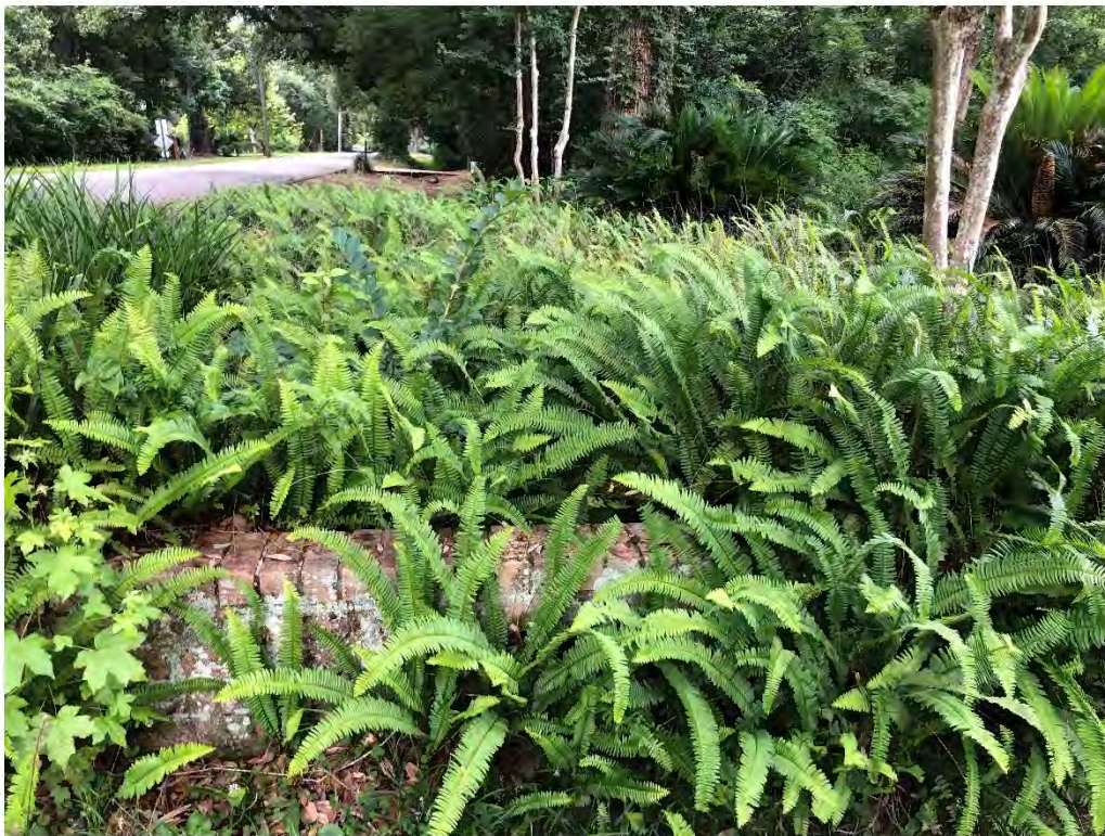
Figure 9150: Photo taken facing West toward an overgrown P-CO-21 along Oak St.
