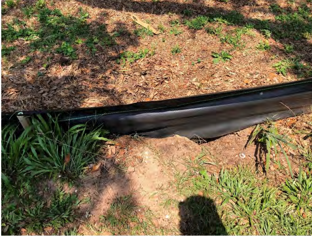
Figure 9625: Photo taken facing West toward a crushed and very silted OAK-CO-6 across Jessamine St.
