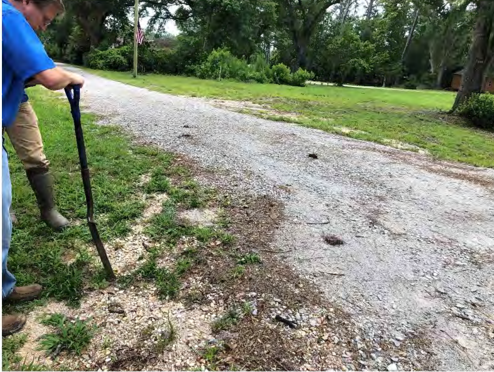
Figure 9098: Photo taken facing South toward a gravel-filled P-CH-29 along Oak St.
