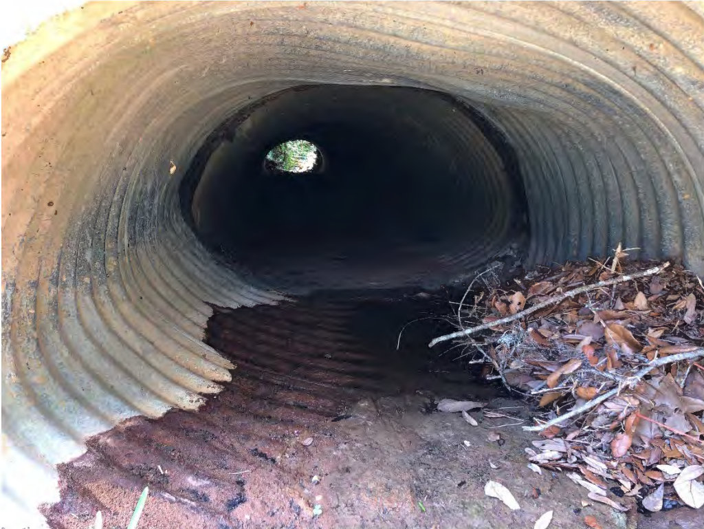
Figure 9109: Photo taken facing West toward a crushed corrugated metal P-CH-28 along Oak St.
