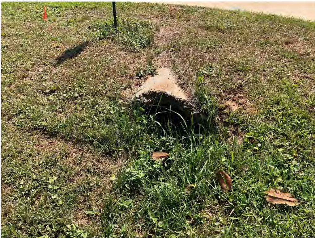
Figure 9577: Photo taken facing West of MN-CO-15 at the intersection of Gates Ave and a driveway.
