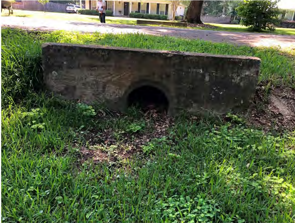
Figure 9508: Photo taken facing East toward VG-CO-7 that crosses Village Green Drive.
