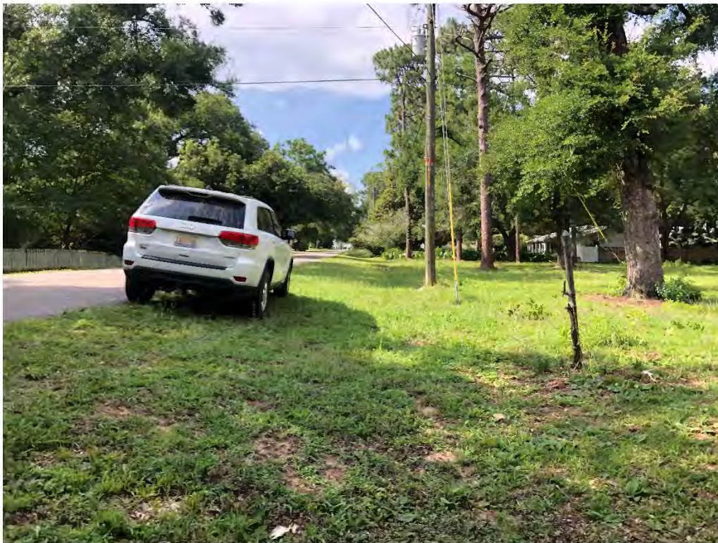
Figure 9239: Photo taken facing North toward a silted P-CH-17 along Pecan Grove St.
