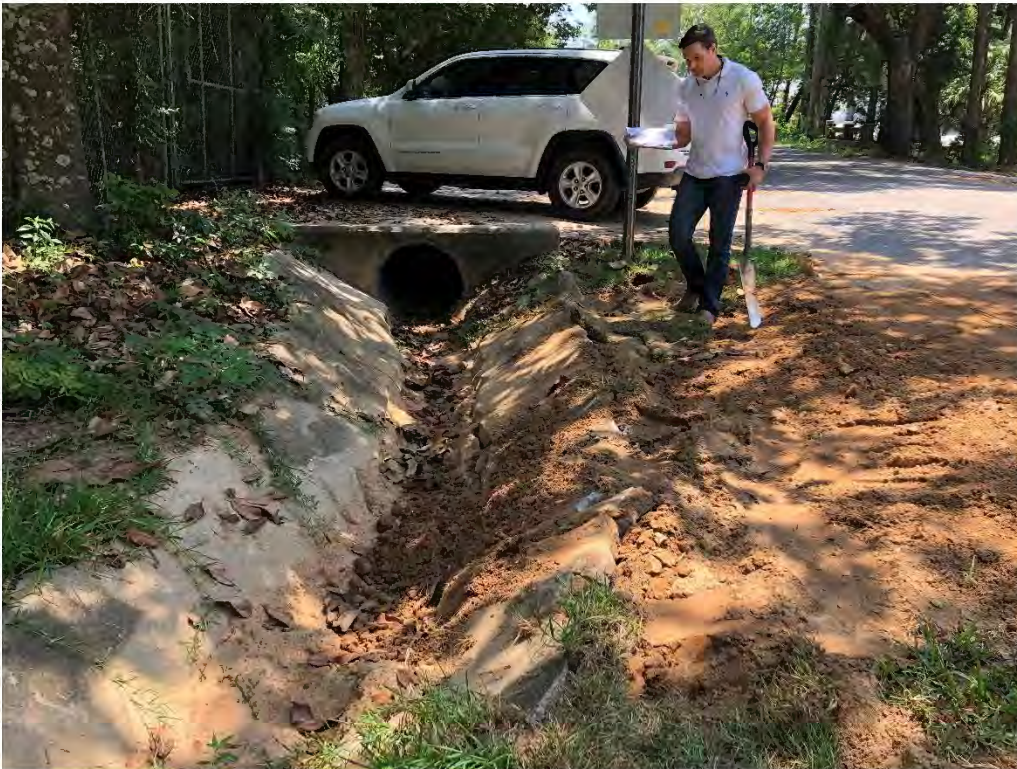
Figure 9662: Photo taken facing NE toward a silted OAK-CO-25 with erosion around the driveway along Oak St.
