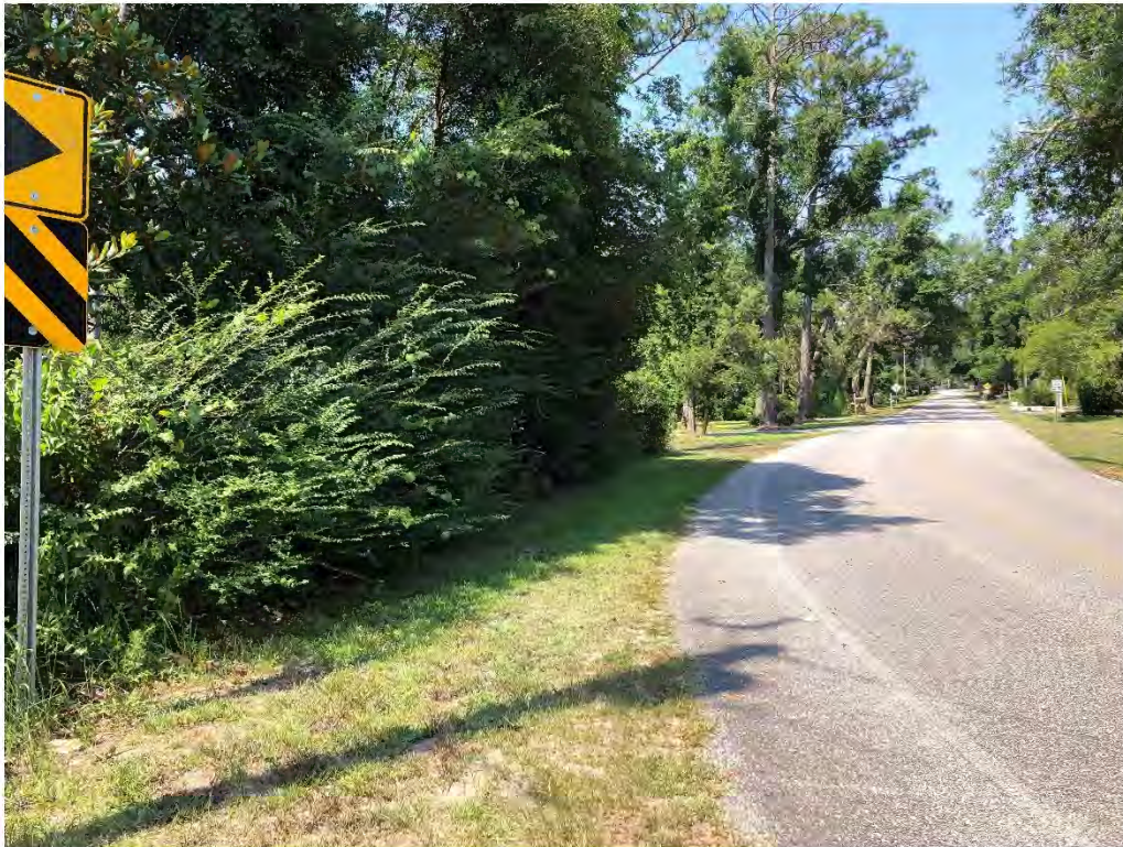
Figure 9560: Photo taken facing SW of MN-CH-12 at the intersection of Old Marlow Road and Gates Ave.
