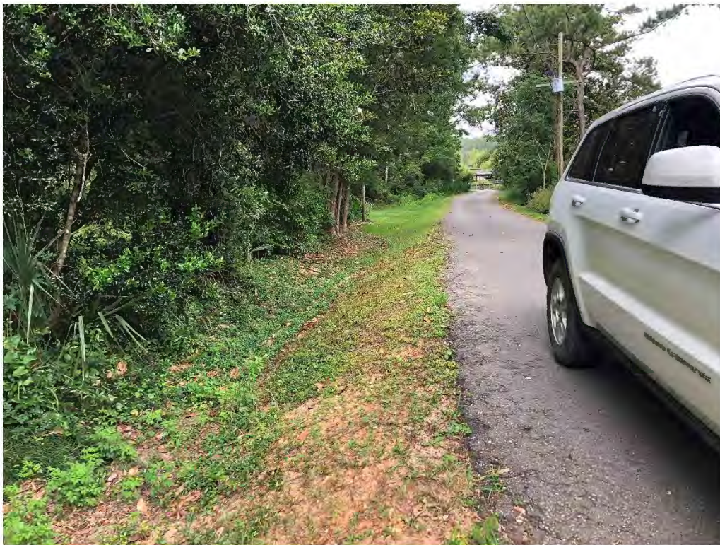
Figure 9181: Photo taken facing South toward BB-CH-13 along Bay St.
