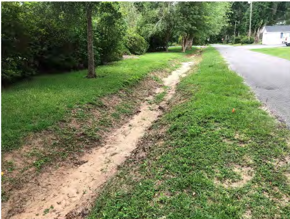
Figure 9190: Photo taken facing South toward BB-CH-10 along Bay St.
