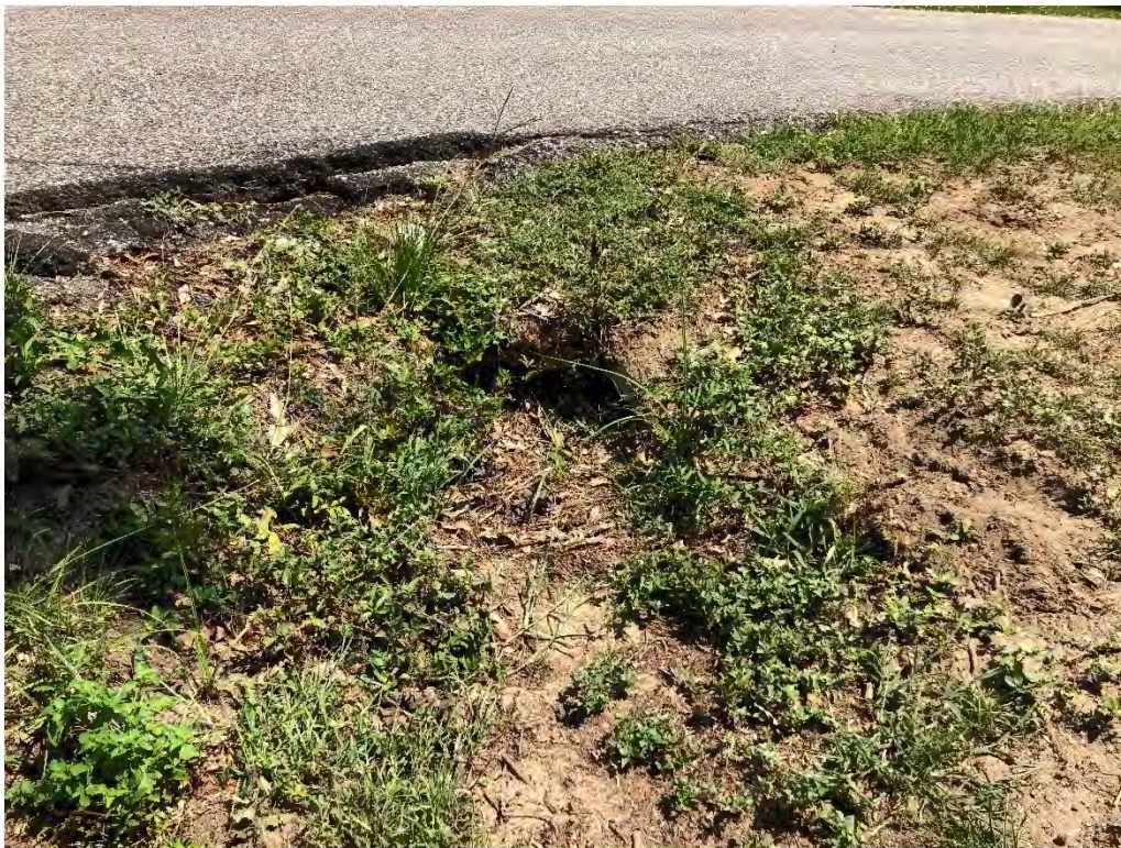
Figure 9594: Photo taken facing North toward MN-CO-7 at the intersection of HWY 49 and School St.
