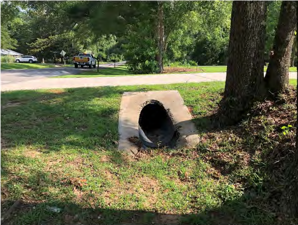
Figure 9267: Photo taken facing South toward P-CO-11 at the intersection of Pecan Grove St and a residential driveway.
