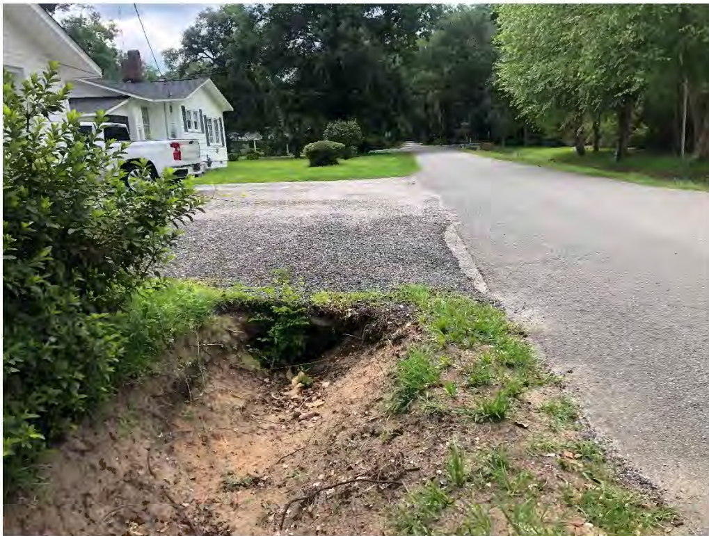
Figure 9184: Photo taken facing North toward BB-CO-9 along Bay St.
