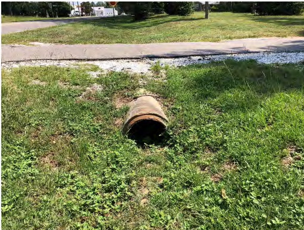
Figure 9614: Photo taken facing North toward a silted MN-CO-3 at the intersection HWY 49 and a driveway.
