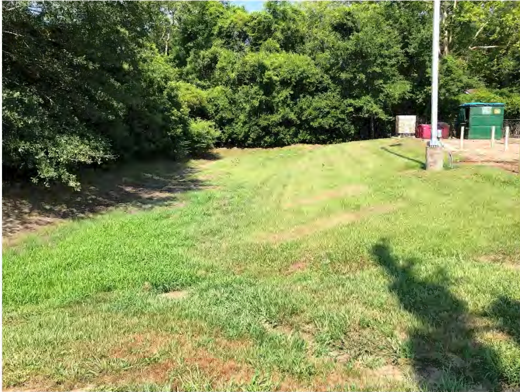
Figure 9532: Photo taken facing West toward a ditch along Magnolia Springs HWY.
