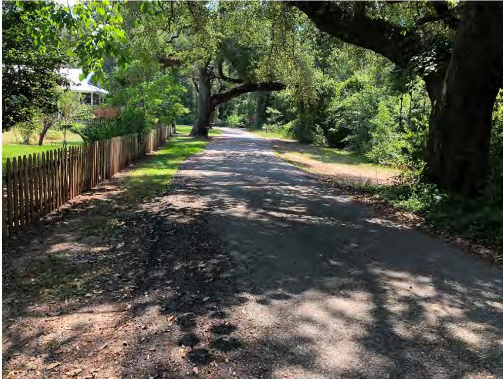
Figure 9647: Photo taken facing East toward a ditch along McCoy Ln.
