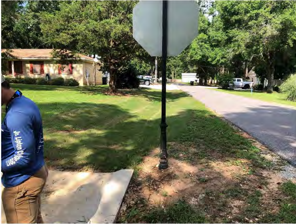
Figure 9259: Photo taken facing North toward P-CH-16 along Pecan Grove St.
