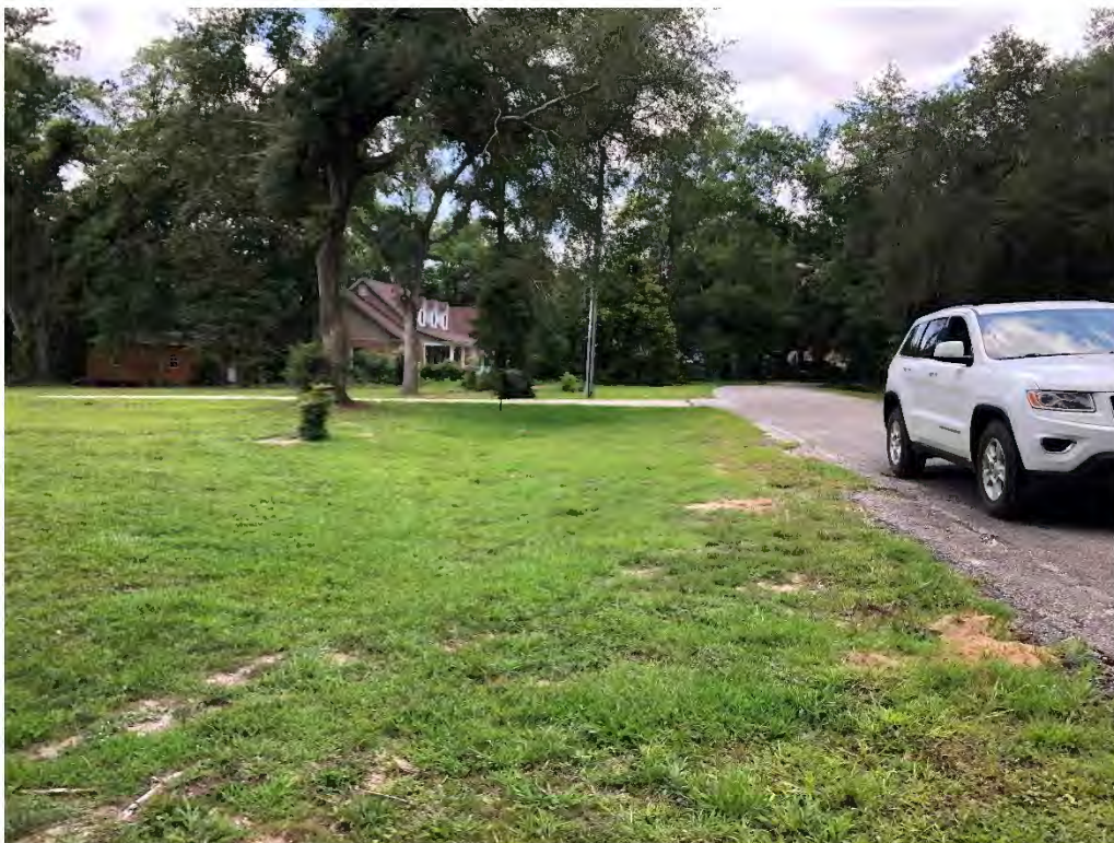
Figure 9091: Photo taken facing West toward a grassed P-CH-Routing-2 along Oak St.
