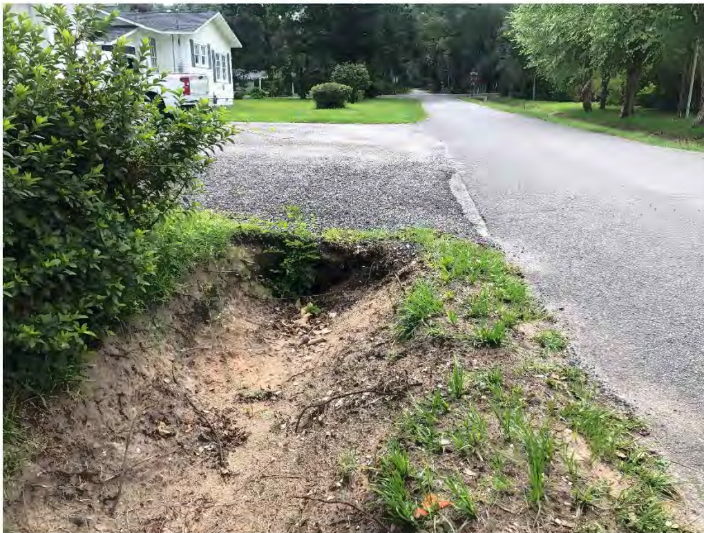
Figure 9187: Photo taken facing North toward BB-CO-9 along Bay St.
