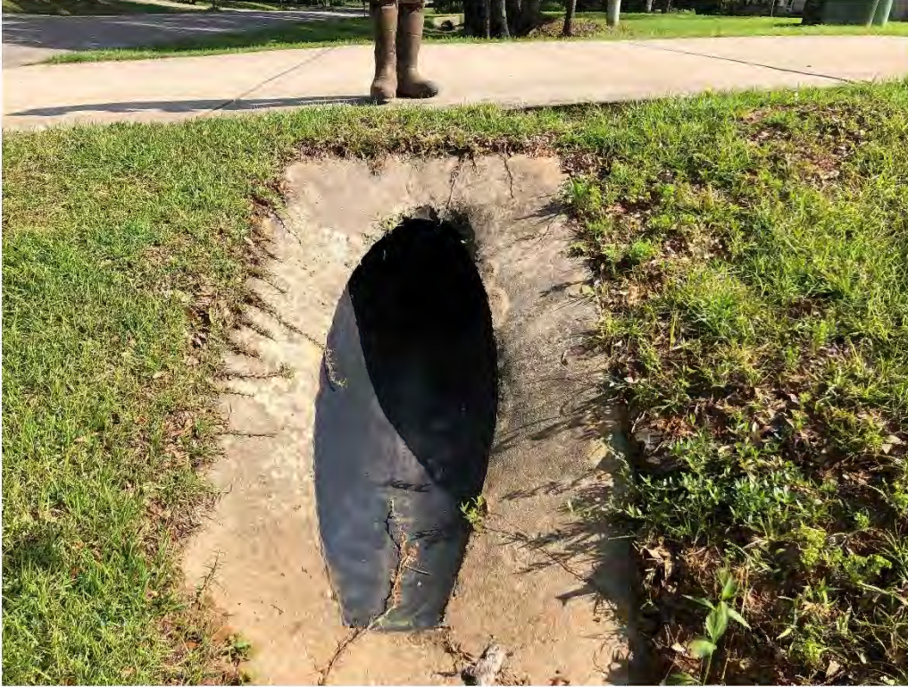
Figure 9271: Photo taken facing North toward P-CO-13 at the intersection of Pecan Grove St and a residential driveway.
