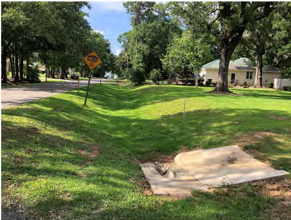
Figure 9258: Photo taken facing North toward P-CH-14 along Pecan Grove St.
