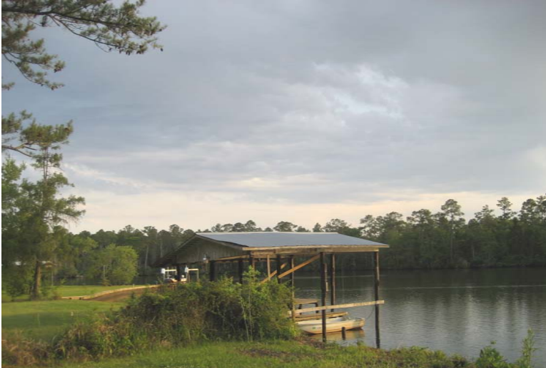
Figure 3-1: Private Properties Facing the Magnolia River Source: Gould Evans
