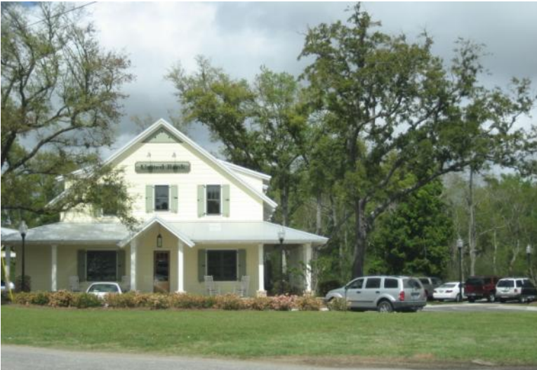
Figure 4-7: United Bank along U.S. Highway 98 Source: Gould Evans
